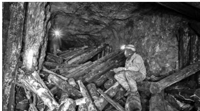
Rescue workers take a break during ongoing attempts to reach three trapped workers at Lily Mine – a rescue mission prolonged by management's profits-before-people attitude
